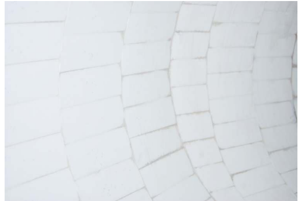
Wedge Type Liner Fitment (Alumina Bend)
